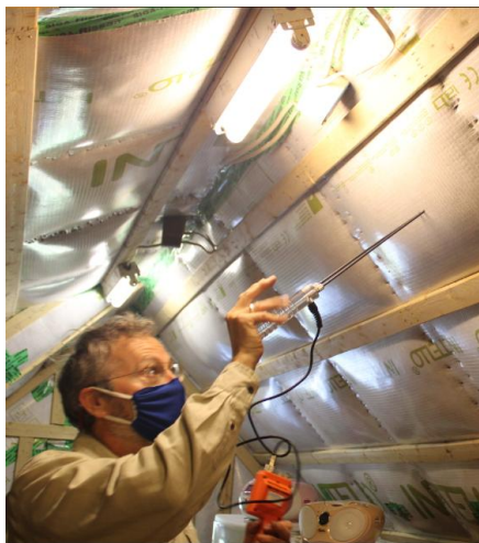
South Roof Slope
